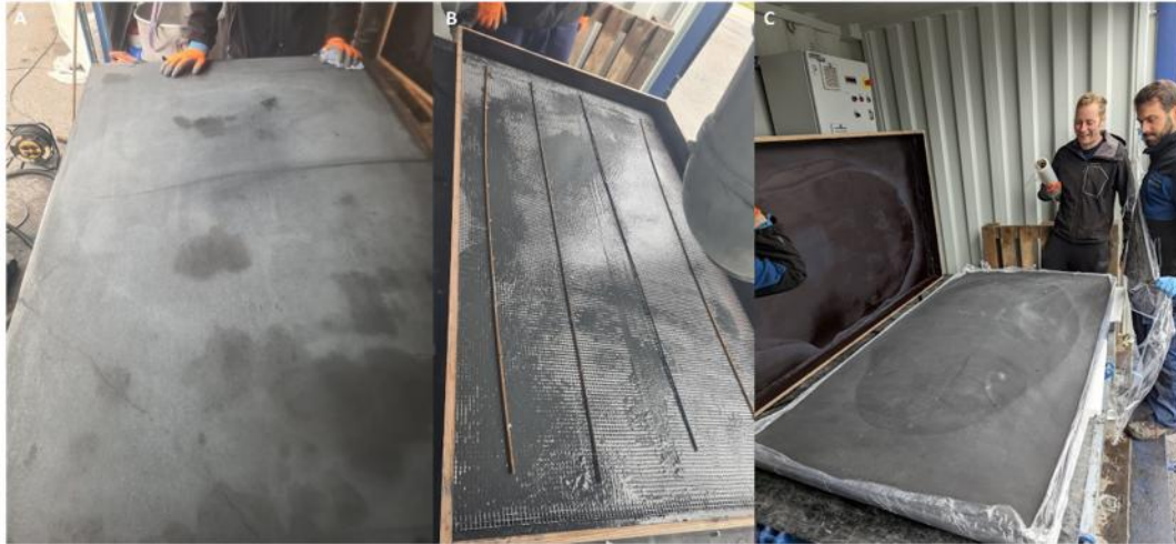
Figure 6. Left: Table top using solely steel fibers as reinforcement, Middle and Right: Production and demolding of table top using glass fibers and steel reinforcement.
