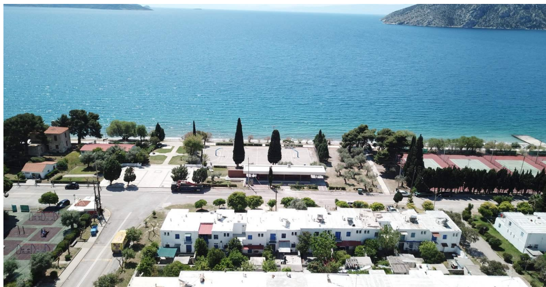
Figure 10: Photos from the finalized House of Bauxite in the Aspra Spitia settlement, Greece.
